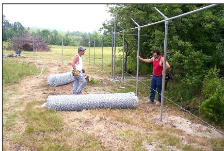
Building one of the 1 st enclosures
